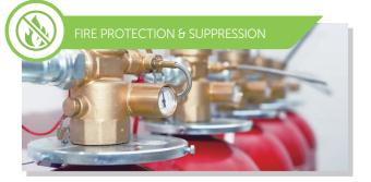
Various fire protection and suppression systems are installed in various regions inside our data centres. Plant rooms and UPS rooms are equipped with Automatic Fire Alarm (AFA) as precautions. Double interlock pre-action sprinkler system, FM-200 or Novec 1230 fire suppression systems are used in data halls for optimal benefits of that particular site.
