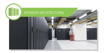
2-hour fireproof wall partitions with all major equipment rooms compartmented in modular design. Data hall with high density zone, raised floor, sophisticated arrangement of Computer Room Air Conditioning (CRAC) units with hot and cold aisle to ensure high cooling efficiency.
