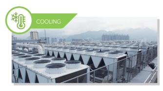
Steady temperature and humidity in data centre are essential. The cooling systems comprise the chiller plants in N+1 configuration fully back up by the generators. Pipes are running through dual risers and ring distribution. CRAC units are dual feed from transformers with Automatic Transfer Switches (ATS).
